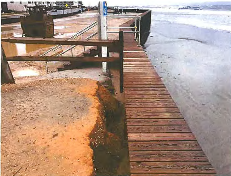
Photo #8 - View of steel bulkhead at 7th Avenue looking northeast showing erosion and flooding on landward side of the bulkhead.
