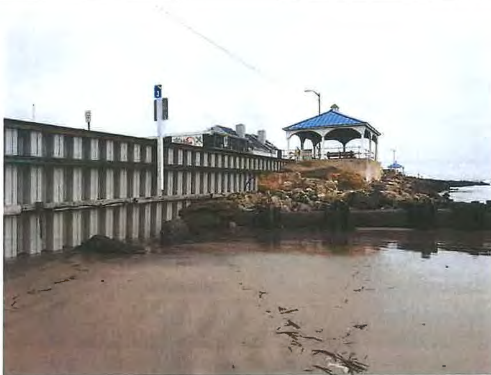
Photo # 2 – View of waterward side of vinyl bulkhead at 3 rd Avenue looking northeast.
