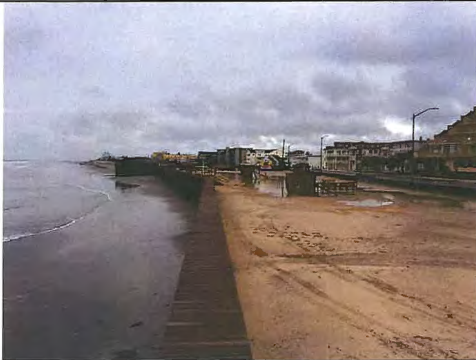
Photo # 7 – View of timber cap and steel bulkhead at 6 th Avenue looking southwest.
